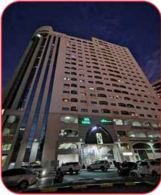
Al Habtoor Tower 1 - Sharjah
